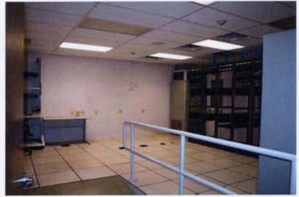
Raised Floor Server Room
