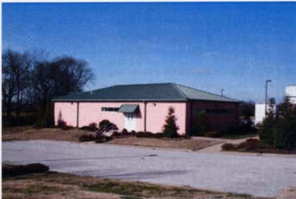
Stand Alone Lab Building
