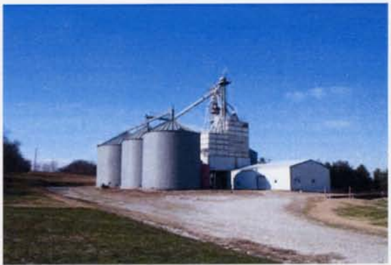
Silos and Storage Warehouse
